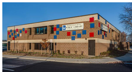
The Hillcrest Heights library opened in this location in 1976; it had been housed in rented space since 1963. PGCMLS
